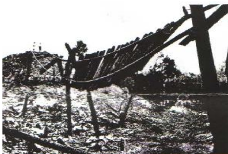
Fire -twisted remains of bridge over Dirty Hollow Creek (photograph in Age April 1965)
